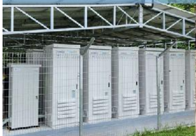
152 kWp PV-DG-BESS Decentralized Microgrid System, Kapas Island, Malaysia
