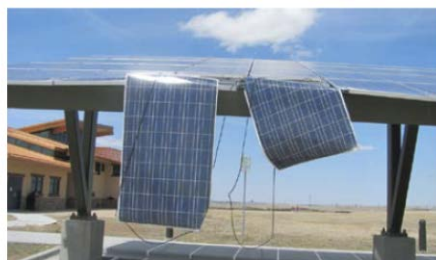
Figure 5: Modules broken by snow load.
