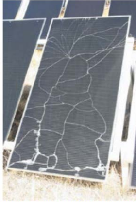
Figure 6: Thin film module with broken front glass.
